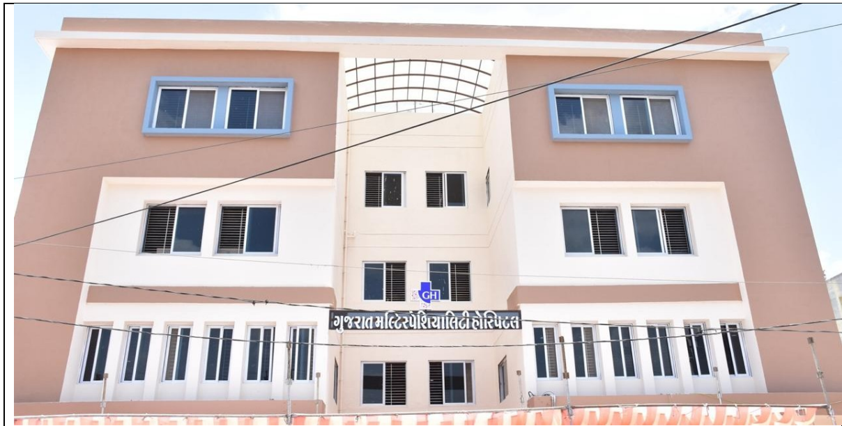
Front view of Gujarat Multispeciality Hospital, Godhra
