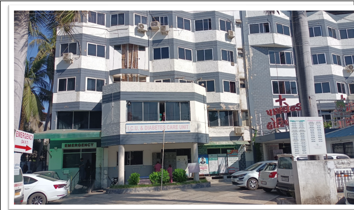
Front view of Raj Palmland Hospital, Bharuch
